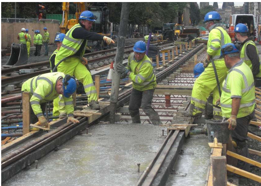
Figure 4-Pouring of Track Concrete Layer, encasing Rheda Trackform, after placement of Track
