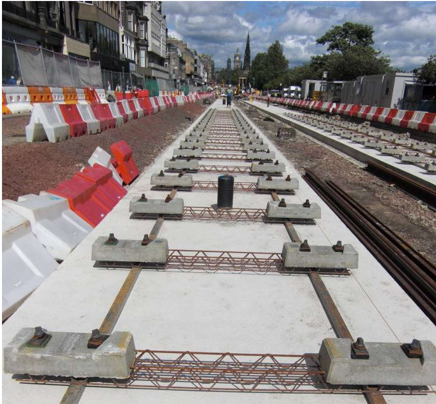
Figure 3-Installation of Rheda Trackform on top of Track Improvement Layer in Princes Street
