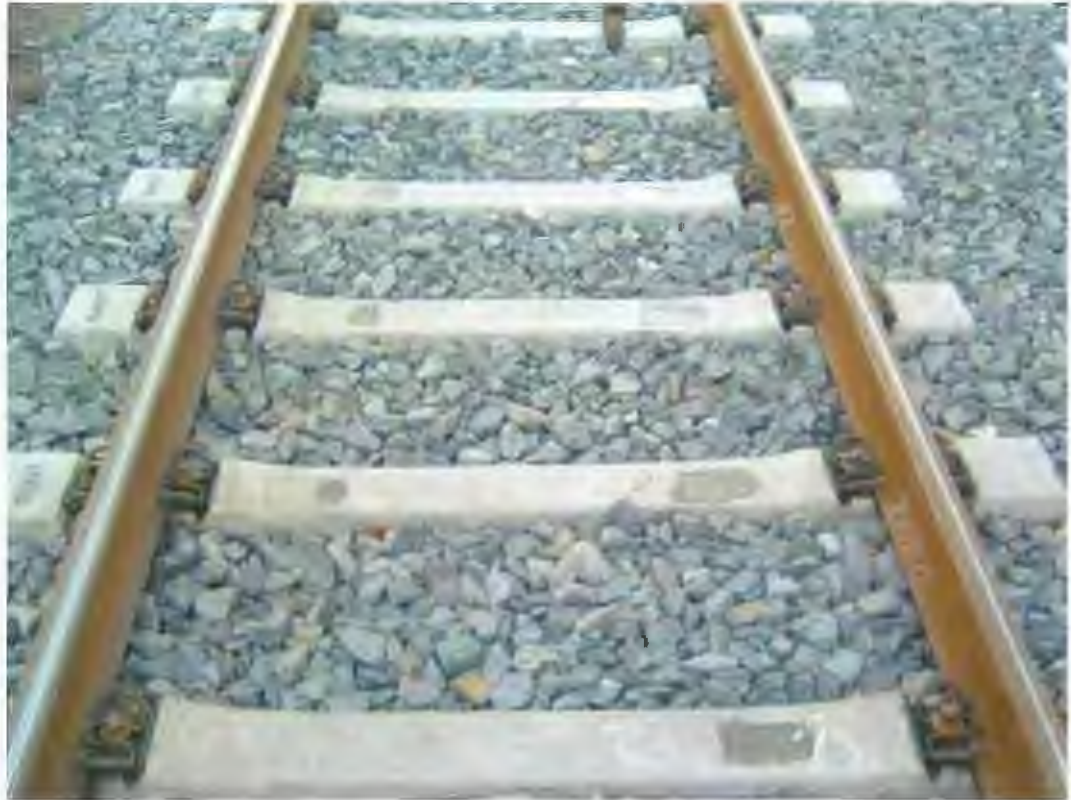
Figure: Example for Ballasted Track
