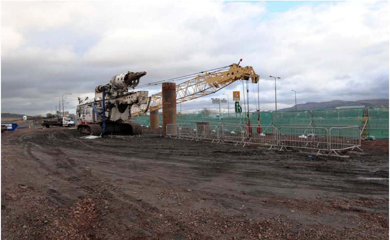
Sect. 5c - Piling Rig 8a Underpass (27/11/08)
