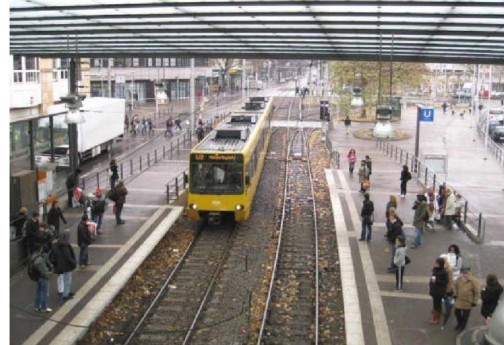
Stuttgart, December 2008: variety of type of alignments on standard-gauge light rail system upgraded from previous metre-gauge street-based tramway
